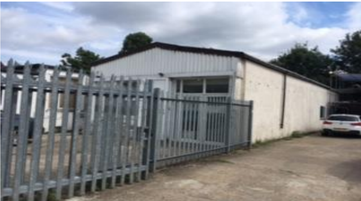
Existing parking around application property
